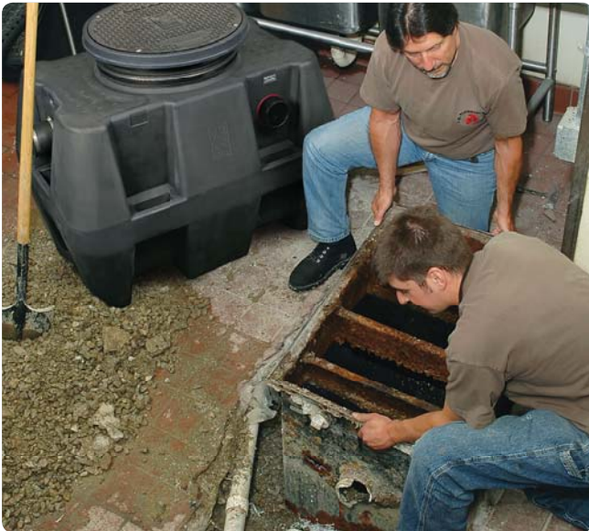
Replacement of rusted steel unit with Schier model GB-75
