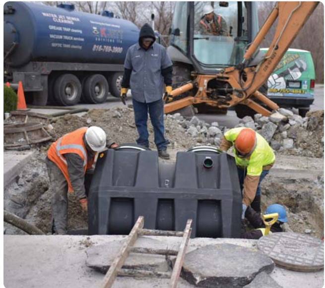
Replacement of corroded concrete unit with Schier model GB-250
